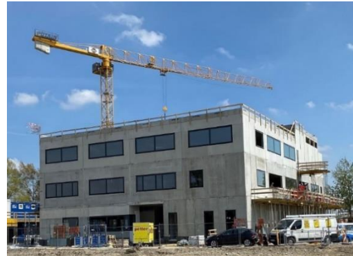
Current Status of Construction Works (May 2021)
